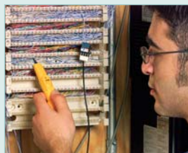
Transmitter injects traceable signal into cables, checks telephone lines, and performs continuity checks
